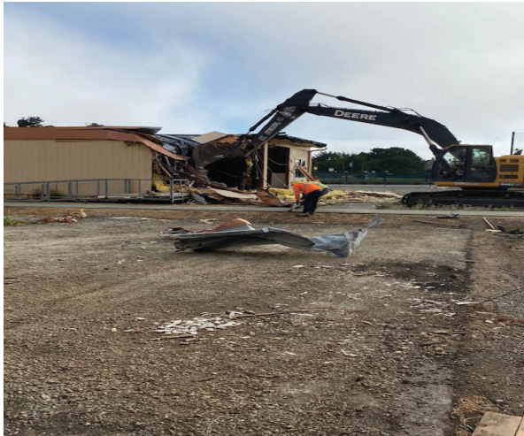
Building 3A-E Portable Replacement Progress
