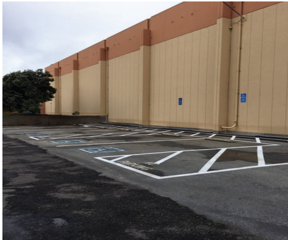
Building 3 South Wall Waterproofing
