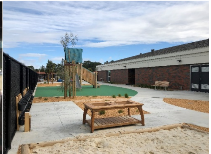
Building 14 Play Yard
