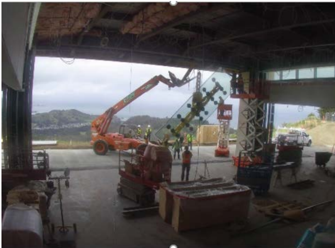
Building 12 Glass Install
