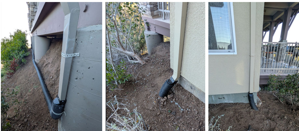
2.3 Completion of the four downspouts connected to the flexible stormwater drainage system.
