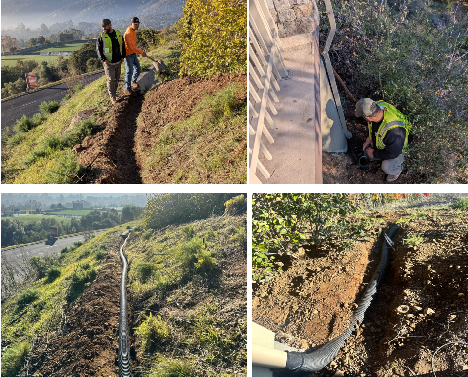
2.2 GBC crew installing the 4-inch flexible drainage pipe system and connecting it to the concrete drainage channel.
