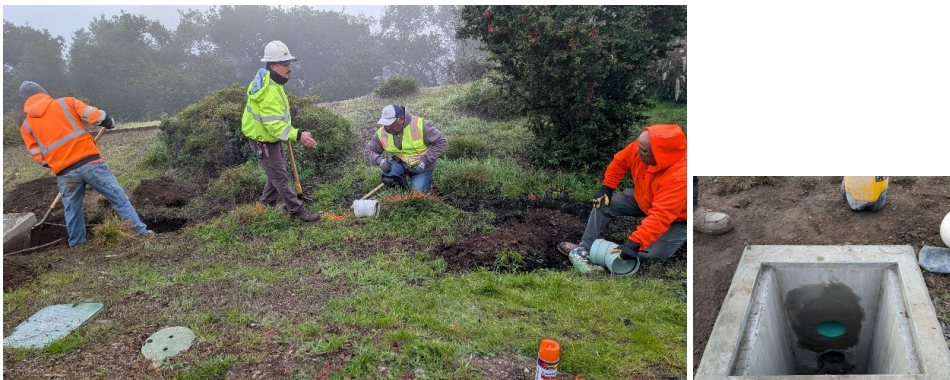
1.2 Golden Bay Construction (GBC) crew rerouting the exposed 6-inch diameter pipe.
