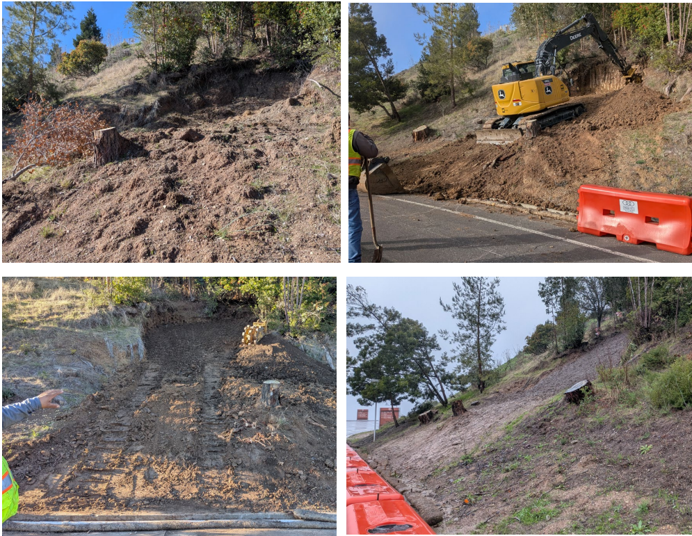
3.1. Eroded area and GBC team working on stabilization measures and final conditions.
