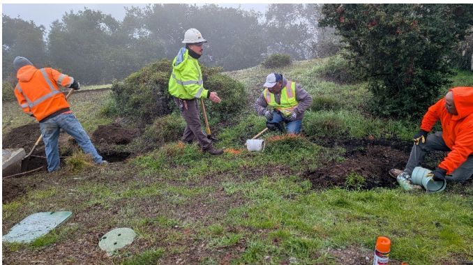
1.2 Golden Bay Construction (GBC) crew rerouting the exposed 6-inch diameter pipe.
