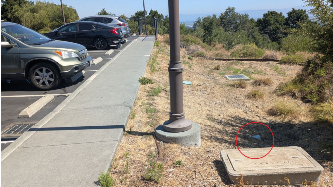
1.1 The Bioretention Area, with an exposed 6-inch diameter pipe highlighted in red.
