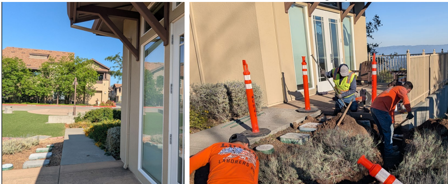
2.5 Downspout discharging onto the exterior deck, with GBC crew installing the stormwater connection pipe system.
